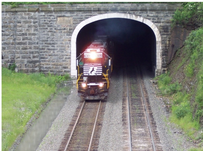
NS 6305 blasting out of the Gallitzin Tunnel after climbing the grade at Horseshoe Curve. Photo by D Chance
