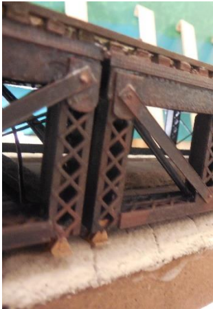
Figure 1 – Bridge shoes are visible where the truss sections meet.
