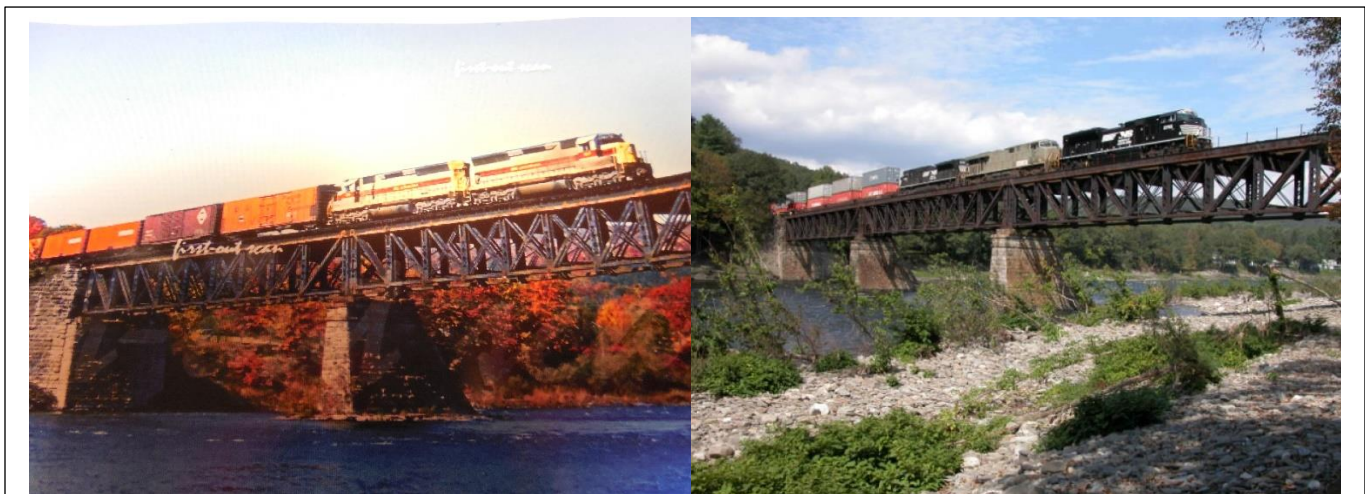
Fig 1 – The Bridge at Mill Rift NY. The left hand photo shows the bridge from Erie days. The Norfolk Southern photo on the right shows that the bridge still stands today. A signature scene for sure.
