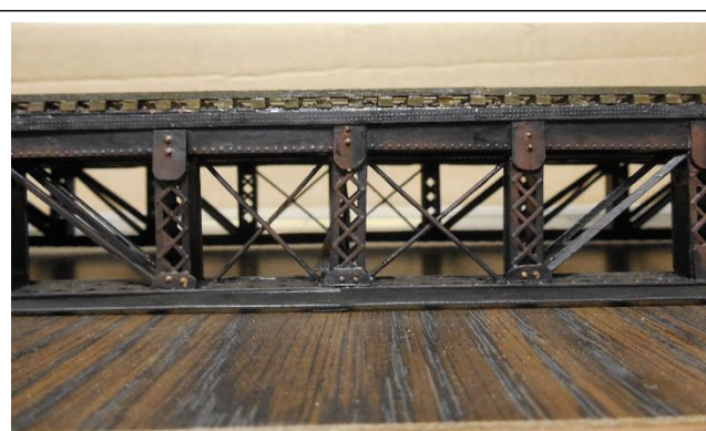
Fig 9 – Gusset plates were installed at junctions of major structural components as per prototype practice.
