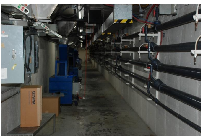
Basement infrastructure distributes electrical, chilled water and air services throughout the building.
