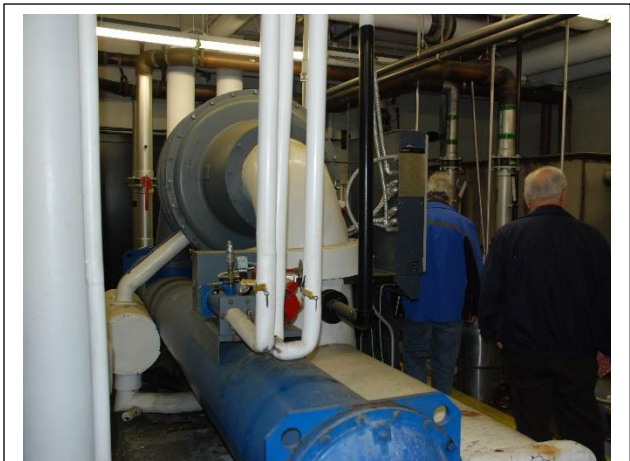
A turbine-style compressor provides air services for the building.
