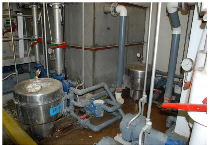
The machinery room provides cooling water and compressed air for all the machines in the production area.
