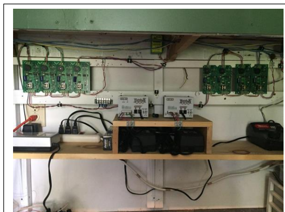
Neat electronics installation can pay off when troubleshooting a problem. Photo by Anthony Perkins
