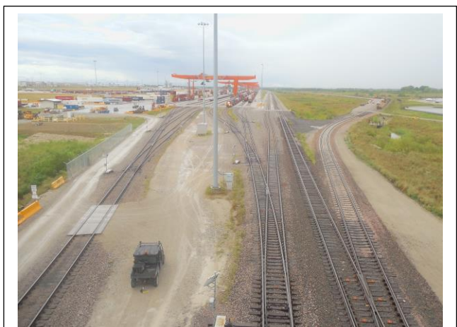
A closer view down the tracks leading into the BNSF intermodal facility.
