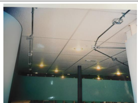
Figure 5 – The lighting conduit installation follows layout contours.
