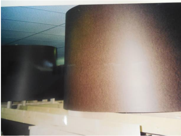
Figure 3 – Backdrops of 1/8" Masonite.
