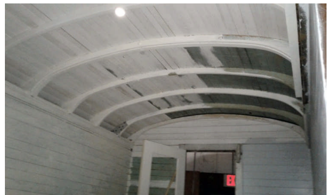
Interior of old baggage car being restored
