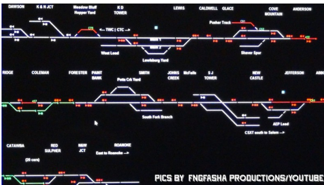
CATS dispatching console
